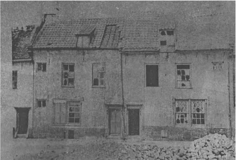
Eighteenth century buildings in Row 118, damaged beyond repair by bombing . Photographed in 1943, prior to demolition.
