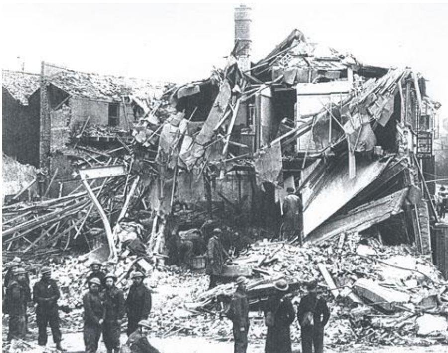
Above: Special Constable's Post in Queens Road
